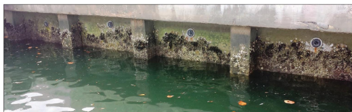
Lake Park Marina in Lake Park, Florida (not shown here), renovated its failing seawall with 150 weep holes from JET Filter. The weep holes relieve hydrostatic pressure behind the wall, providing a mechanism for water to drain through the seawall.
