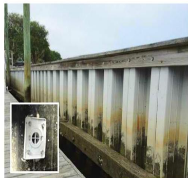
Inlet Watch Yacht Club has approximately 280 weep hole filters by Jet Filter Systems that drain water from behind the retaining wall.
